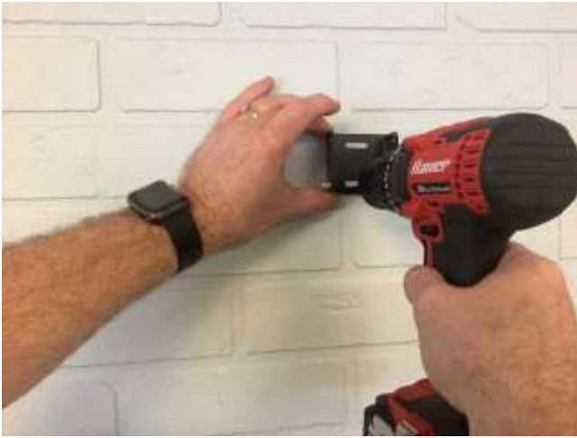
Step 2 – attach bracket to wall
