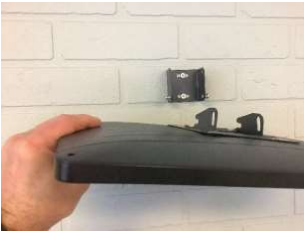
Step 3 – place monitor bracket “hooks” on the bottom screws
