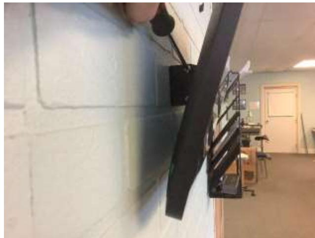
Step 4 – tighten top screws
