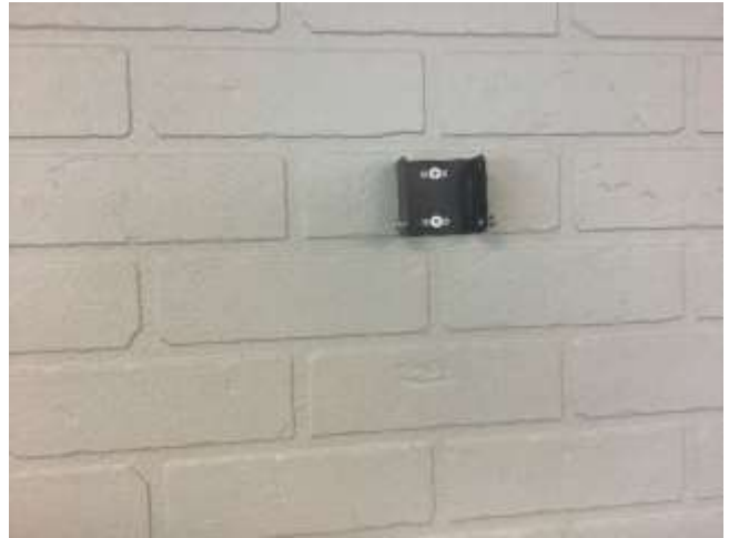
Step 2 – attach bracket to wall
